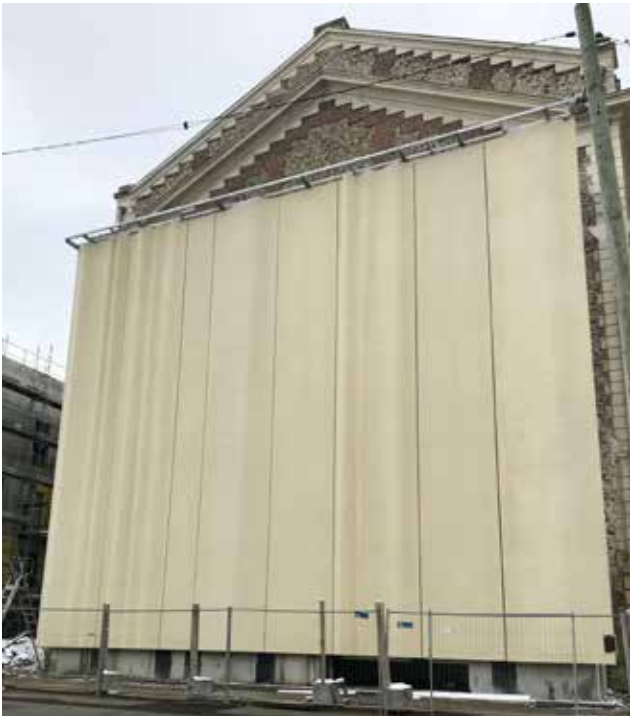
HPC facade of Evreux Theatre in France.
