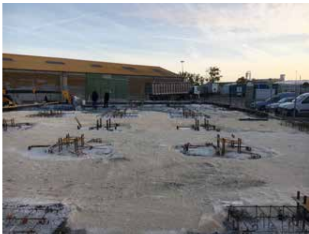
Construction of terminal foundations.
