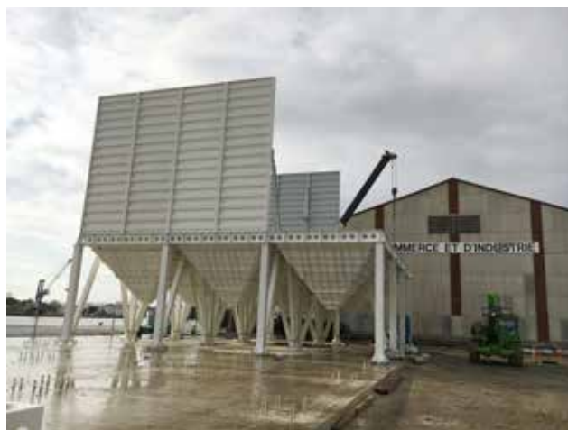
Installation of cement silos.
