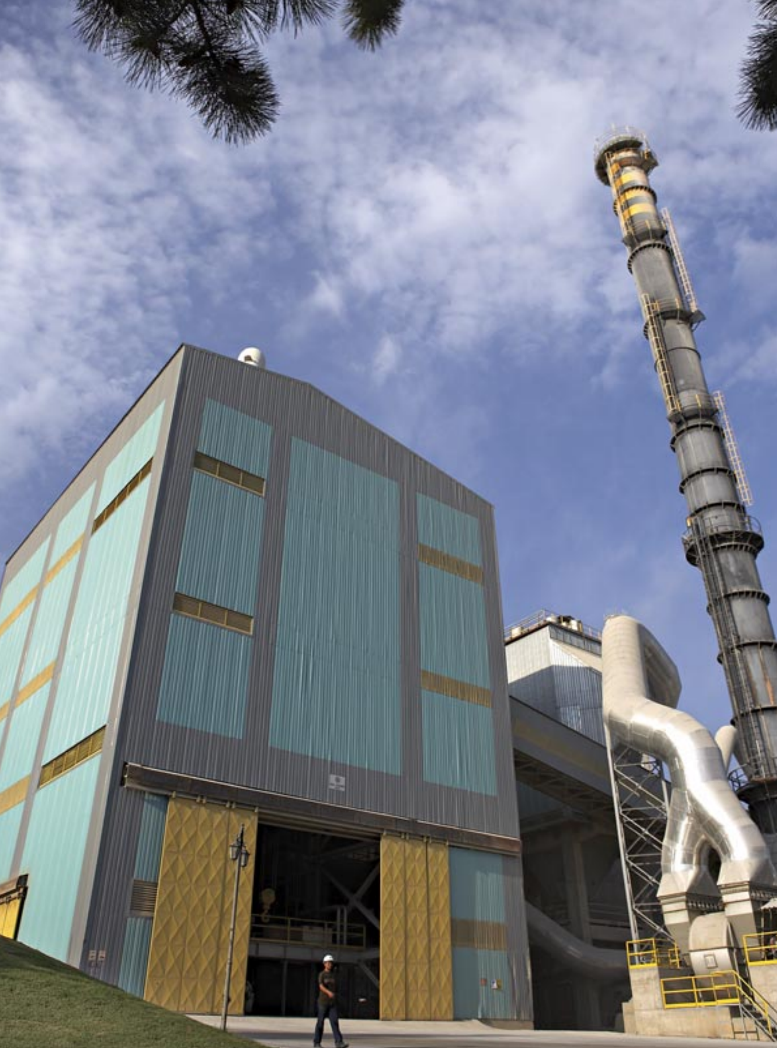
Cement plant in Elazig, Turkey
