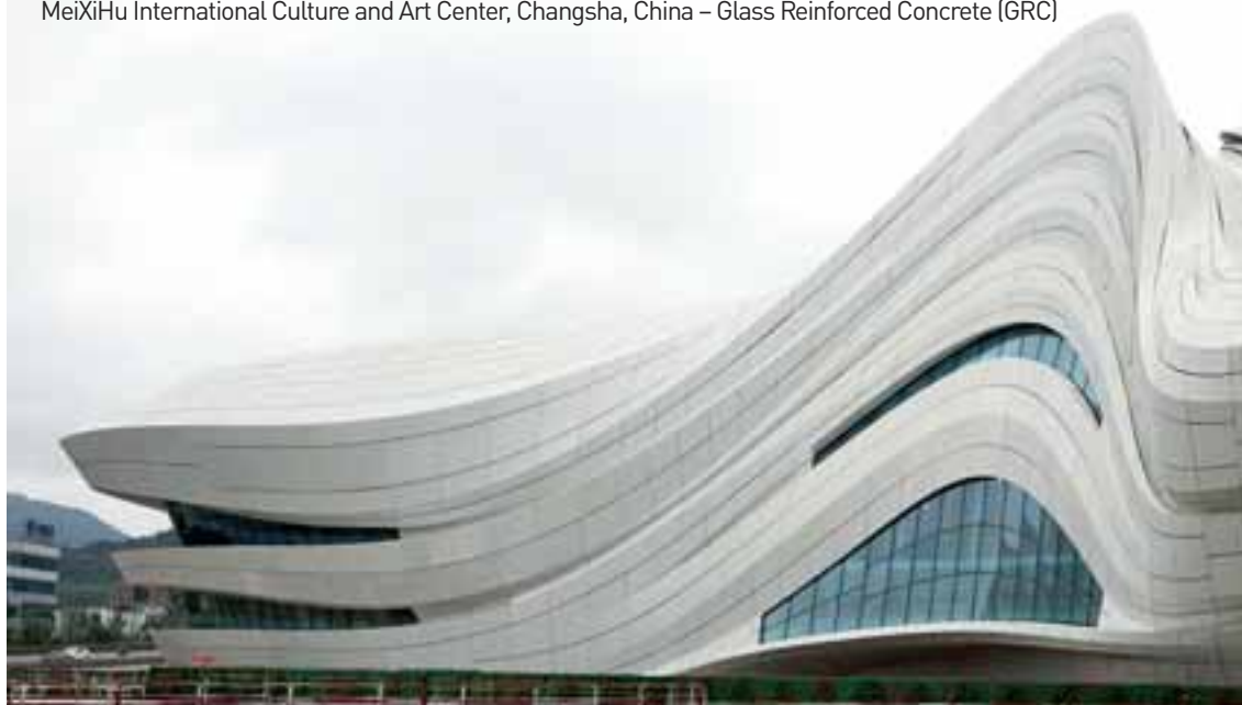
MeiXiHu International Culture and Art Center, Changsha, China – Glass Reinforced Concrete (GRC)
