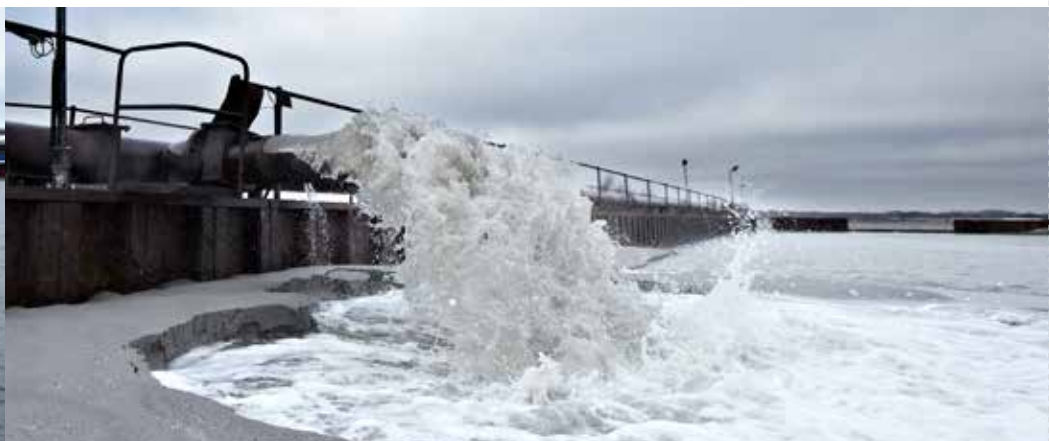
Sand from navigation channels pumped from dredgers to drainage basins ashore
