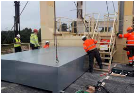
Section 1: First stage, September 2018
