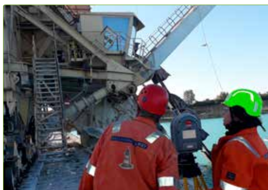
Surveyors preparing the 3D laser scanning of the deep-excavator
