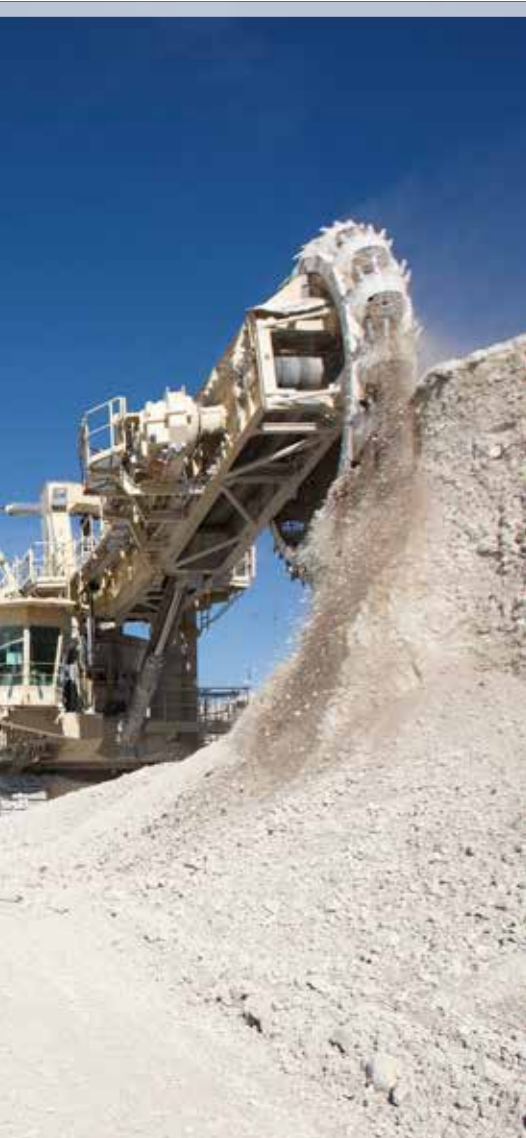
Bucket wheel excavator in the chalk pit
