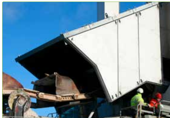
Craning of baffle plates
