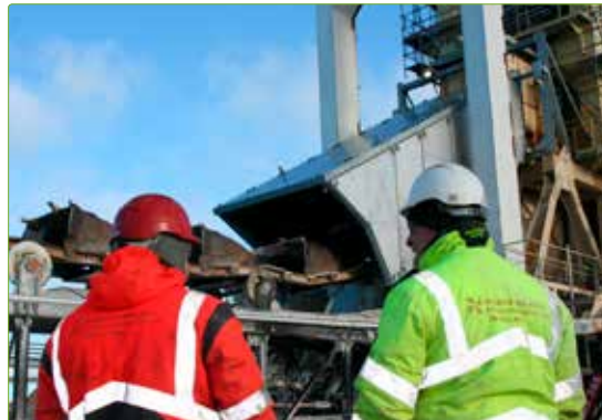
Section 2: Installation in winter, February 2019
