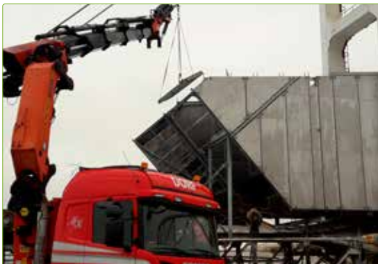
Installation using mobile lift
