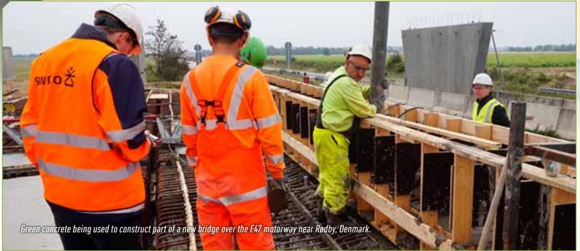
*Green concrete being used to construct part of a new bridge over the E47 motorway near Rodby, Denmark.*
